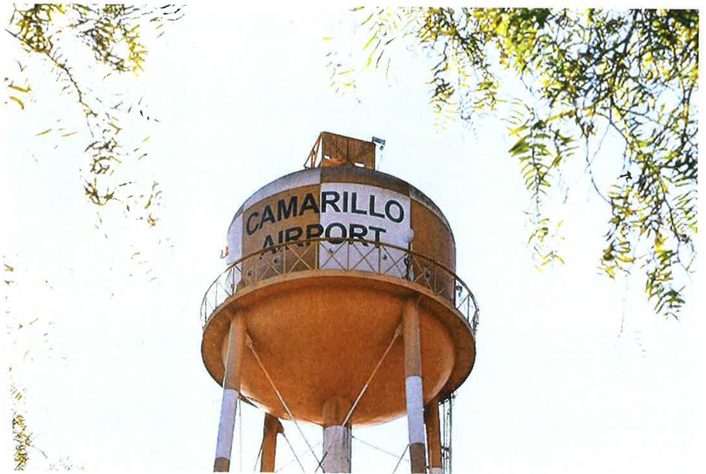
An old water tower is still in use as an airport beacon. (Caroline Sheen)
