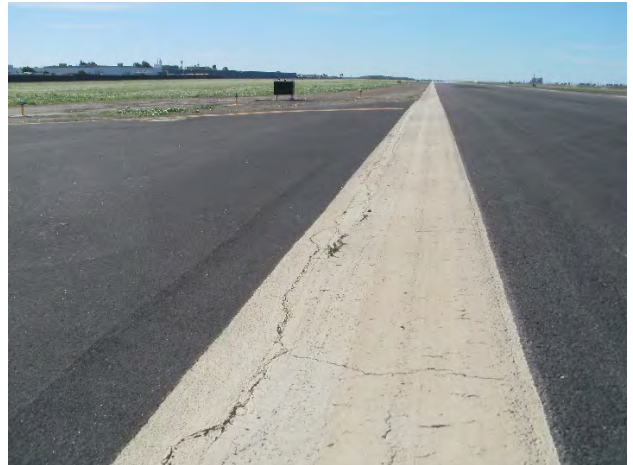
Photo 8: Runway 7-25 Longitudinal Cracking
