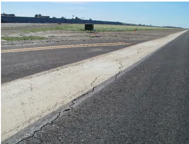
Photo 9: Runway 7-25 Longitudinal Cracking
