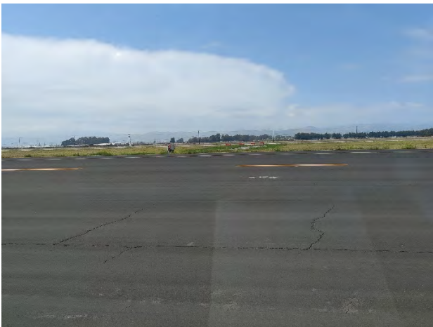
Photo 21: Taxiway F Longitudinal Cracking
