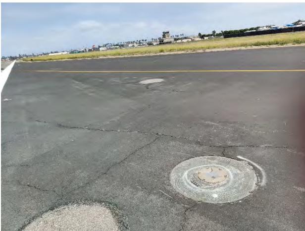
Photo 15: Runway Edge In-Pavement Lights
