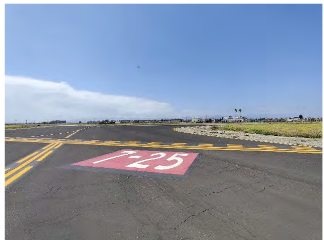
Photo 18: Taxiway C Alligator Cracking
