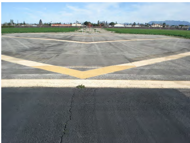
Photo 5: Blast Pad and MALSF System
