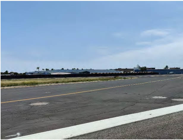
Photo 19: Taxiway D Block Cracking
