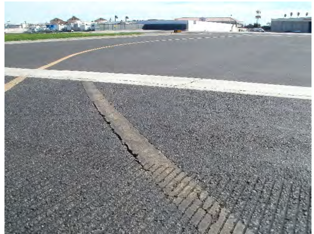
Photo 2: Runway 7-25 Asphalt Scarification
