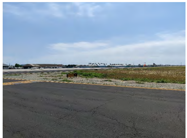
Photo 14: Taxiway A Block Cracking
