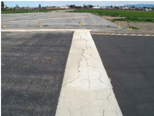
Photo 3: Runway 7-25 Longitudinal Cracking
