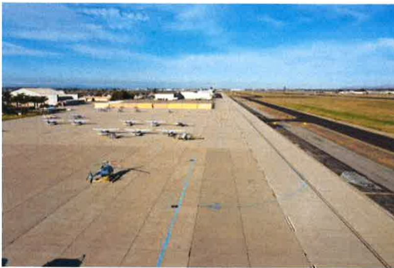
Taxiways at Camarillo Airport. Photo submitted
